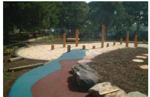
Net play equipment in construction
