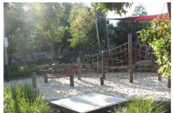
Completed net play equipment
